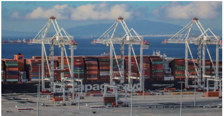
자료: Port Technology(2021.01.18.), https://www.porttechnology.org/news/new-tanger-alliance-terminal-fully-operational-after-receiving-first-vessel/ (2021.01.24. 검색)
