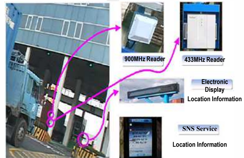
[RFID Gate – Export equipment installed]
